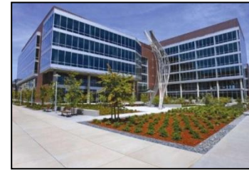
500 Terry A. Francois Blvd
